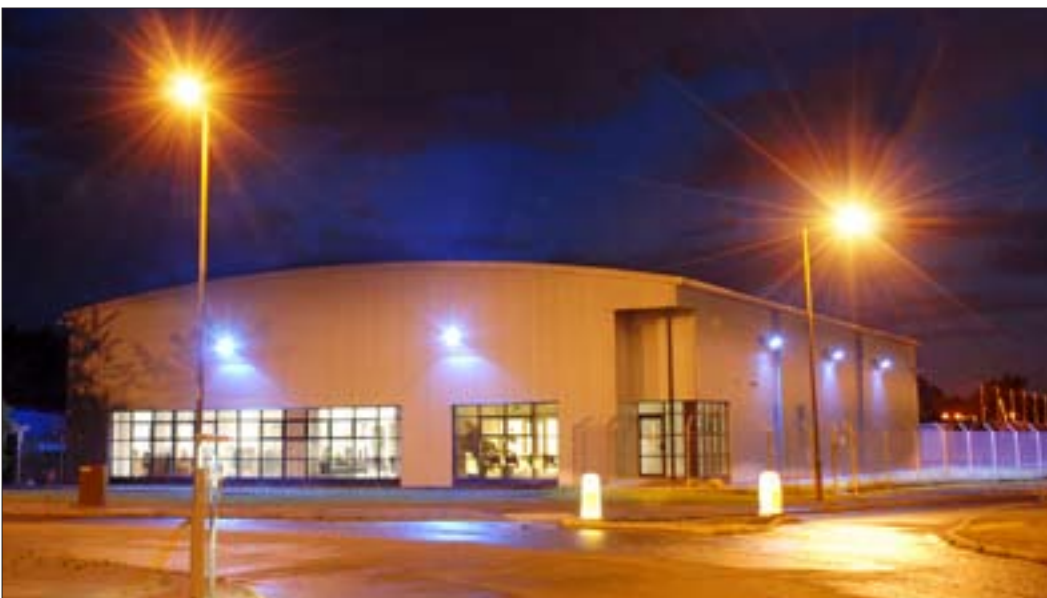
ISP Lumison's Croydon facility
